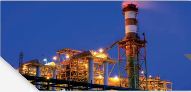
Gaz ve Petrol Gas and Petroleum
