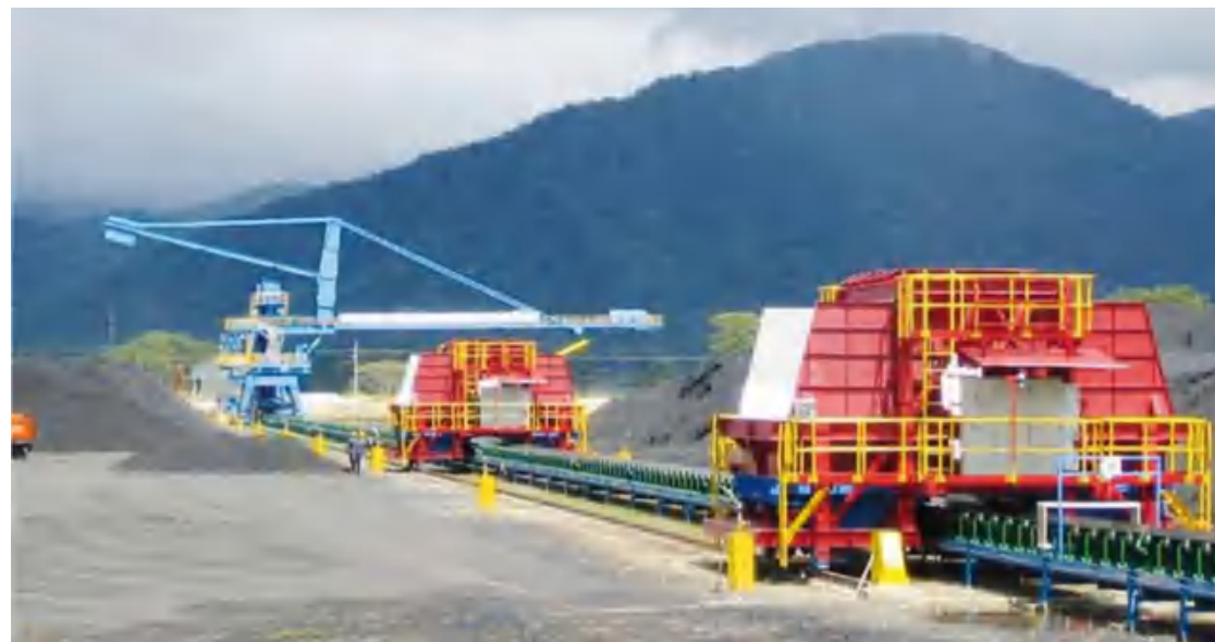
Mineral deposits conveyor
