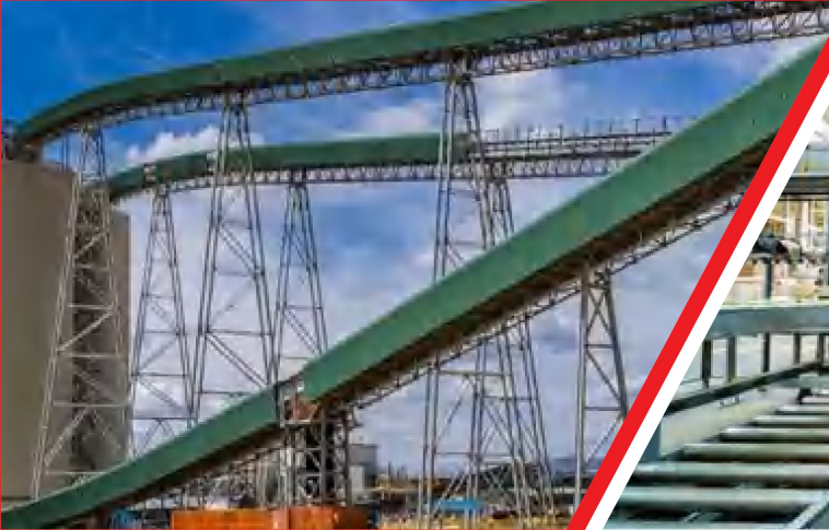
MADEN TESİSİ MINING PLANT
